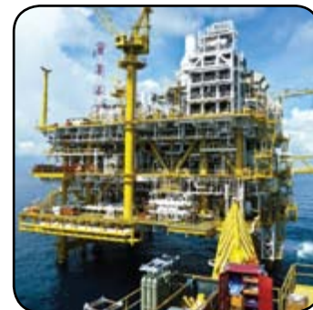
Offshore Platforms & Rigs
