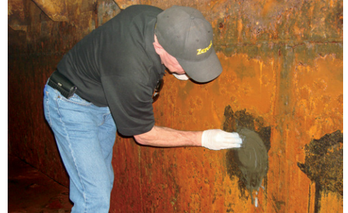
ZERUST® corrosion engineer in the field demonstrating a rust remover
